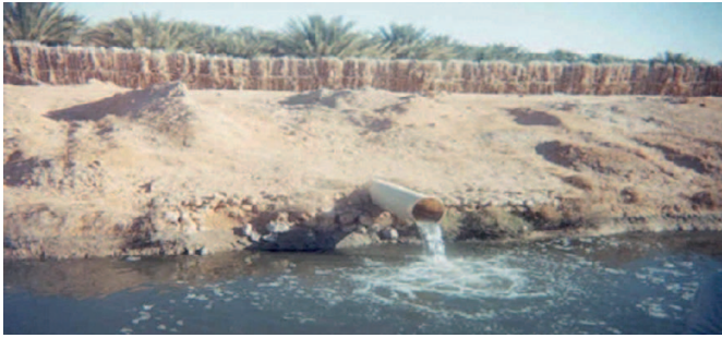
Photo 1: Wastewater spill near the palm plantations.
